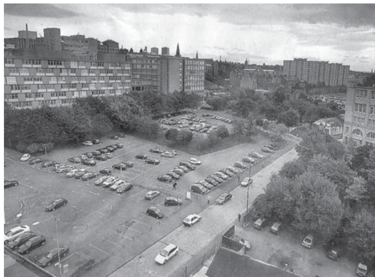
Albion Street City Centre site in Glasgow (H2 Oct 00)
