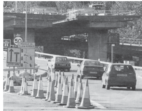
End of the Motorway? This structure is now unlikely to be incorporated in revised plans for the M74 Corridor. Evening Times 28 Sept.
