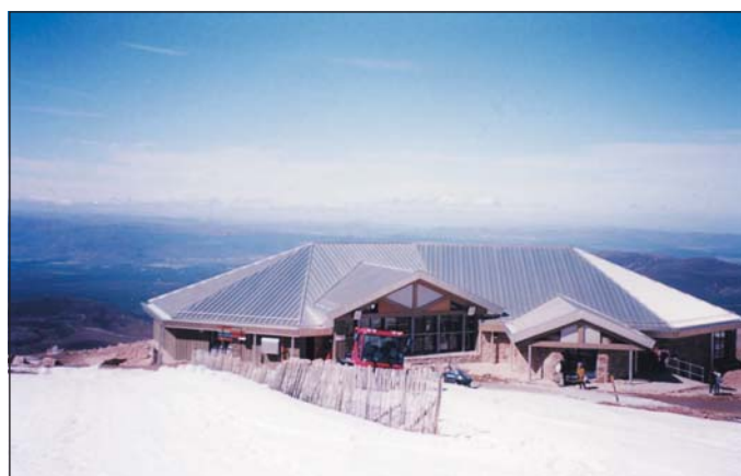
Ptarmigan Top Station and Restaurant / Shop. The Funicular approaches this in a cut-and-cover tunnel.
